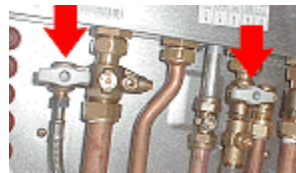
(Fig.2) Integral Filling Valve usually on underside of boiler
