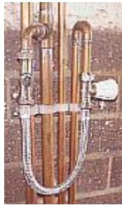
(Fig.1) External Filling Loop
